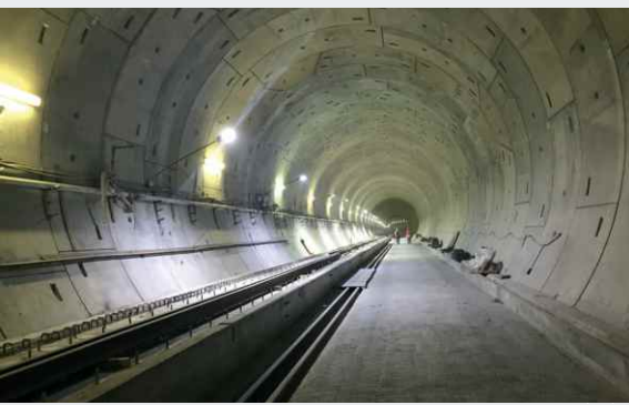
Tunnel ready for installation
