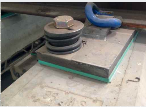
Baseplate pads for VAE turnouts
