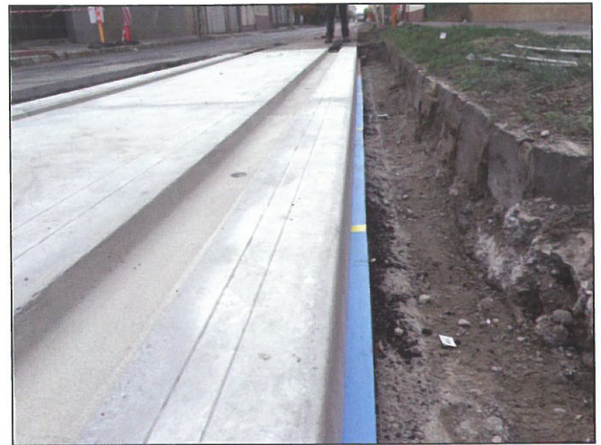
Fig. 4: Concrete slabs with rail channel
