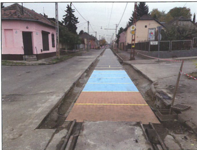
Fig. 2: Transition zone with Sylomer® mats
