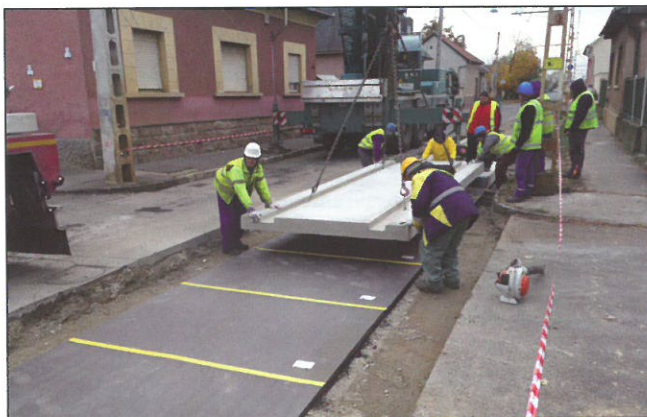
Fig. 3: Installation of the concrete slabs
