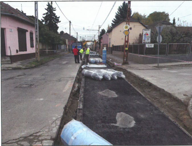
Fig. 1: Initial construction phase of the test section
