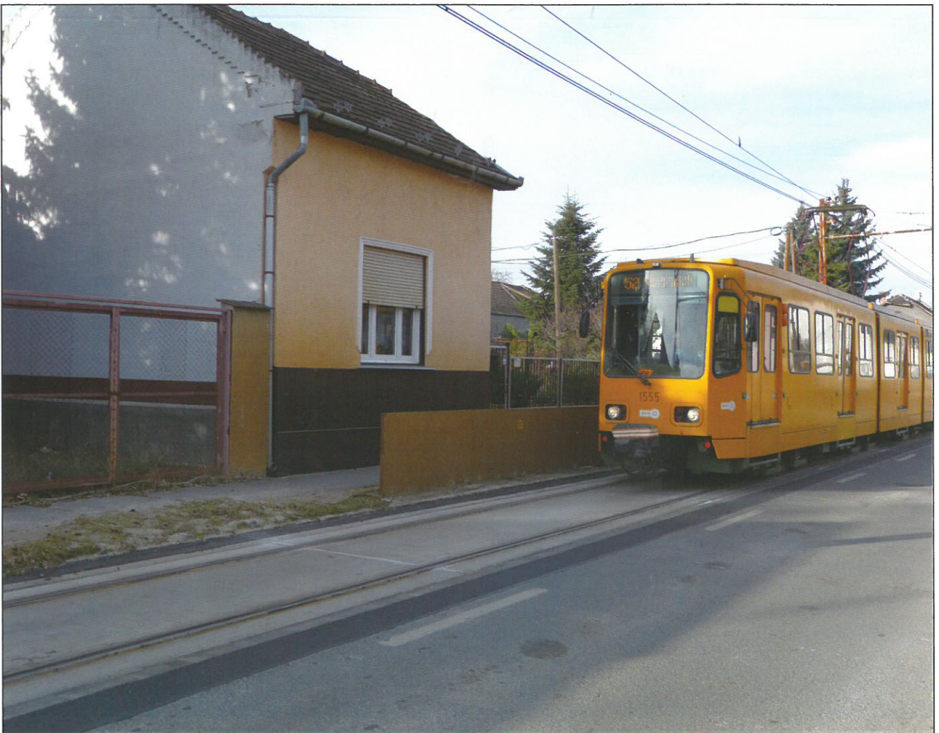
Fig. 6: A T6000 tram passing over the new slab track mass-spring system
