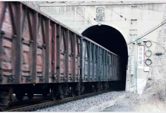
Transition from open track into a tunnel
