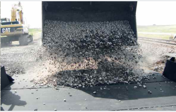
Installation of under ballast mats on a bridge in the USA
