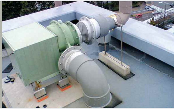
Damping vibrations efficiently: decoupling pumps and pipework
