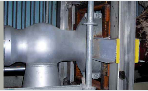
Noise and vibrations are reduced by the elastic decoupling of pumps
