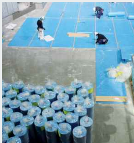
Laying the first layer of Sylomer®
