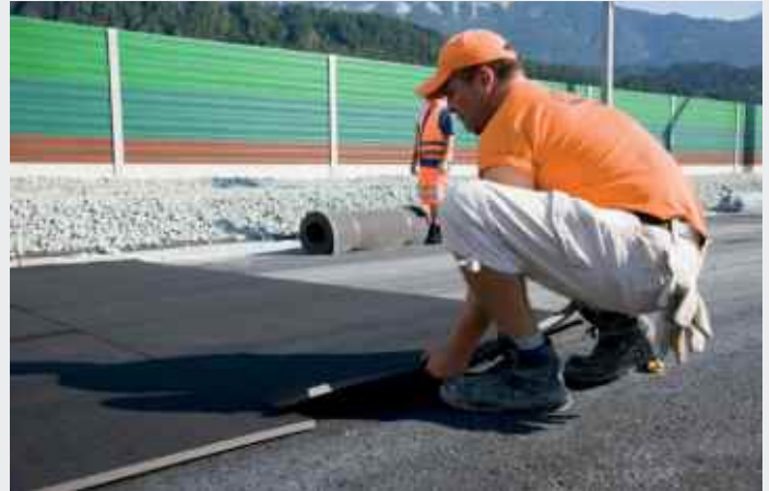
Installation of under ballast mats
