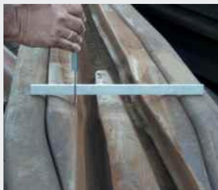
Damage to rails and the turnout frog
