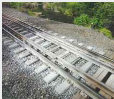
Inhomogeneous load distribution in the turnout causes ballast wear and “white spots”.
