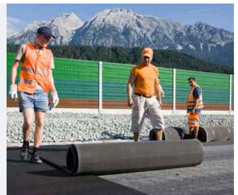
Installation of under ballast mats
