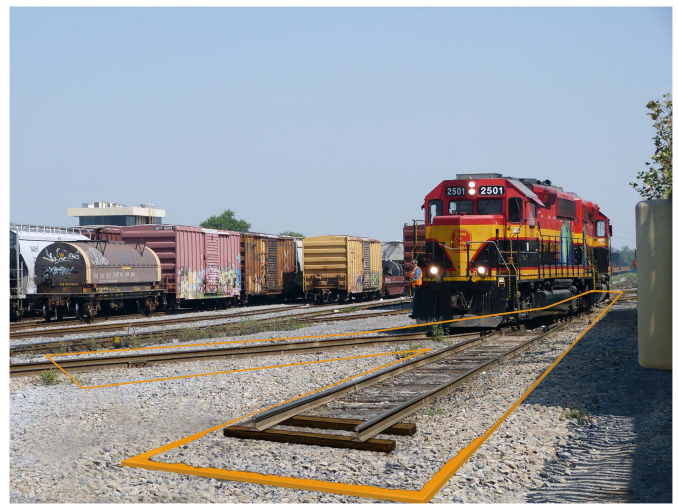
Fig. 9. Location of the UBM in the renovated railroad section. Outlines mark the area equipped with the USM Syldyn DN1019, and the sketched cross section of the superstructure illustrates the UBM's position beneath the ballast [cf. Fig. 5(b)].
