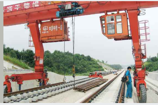
Slab track construction in China
