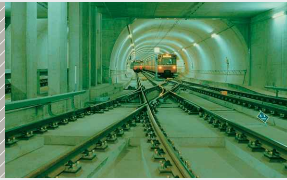
Elastically supported urban railway turnout
