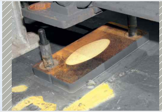
Removing of baseplate pads at London Underground network
