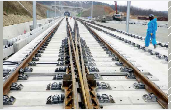
Elastically supported fastening system in high-speed turnout, South Korea
