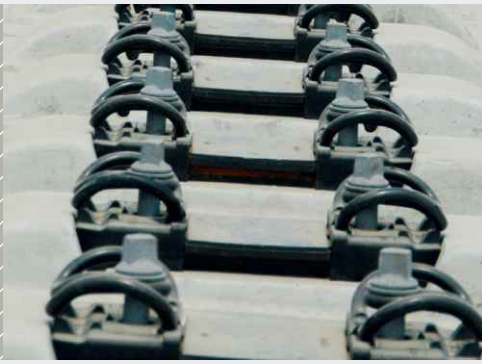
High-speed rail fastening system during assembly
