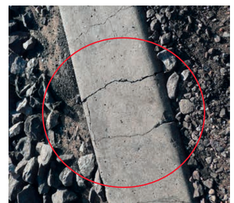
FIG. 8: Examples of typical problems encountered on heavy-haul railway lines throughout the world: destruction of ballast under concrete sleepers (left), fractured tensioning clamps (middle) and cracked sleepers (right) are mostly the result of excessively high dynamic loads
