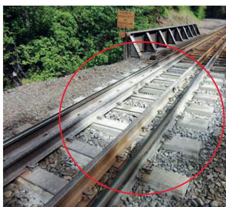
FIG. 8: Examples of typical problems encountered on heavy-haul railway lines throughout the world: destruction of ballast under concrete sleepers (left), fractured tensioning clamps (middle) and cracked sleepers (right) are mostly the result of excessively high dynamic loads
