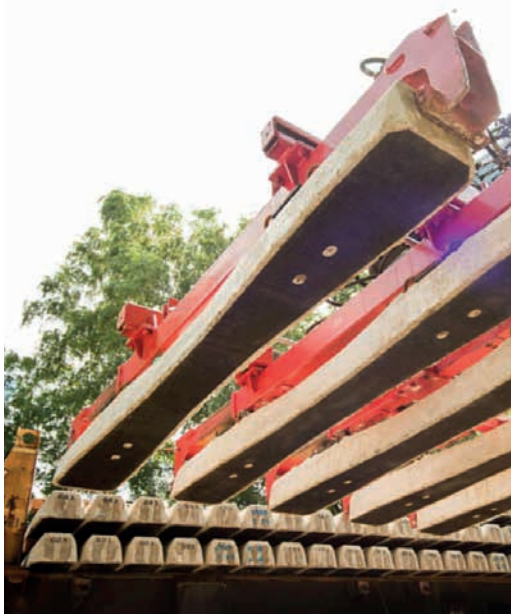
FIG. 9: Laying sleepers with pads
