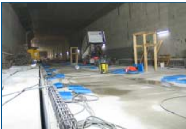
ABOVE LEFT: Sylomer mats were installed in the transition areas to adjust the track stiffness between the rigid and resiliently-mounted track slabs
