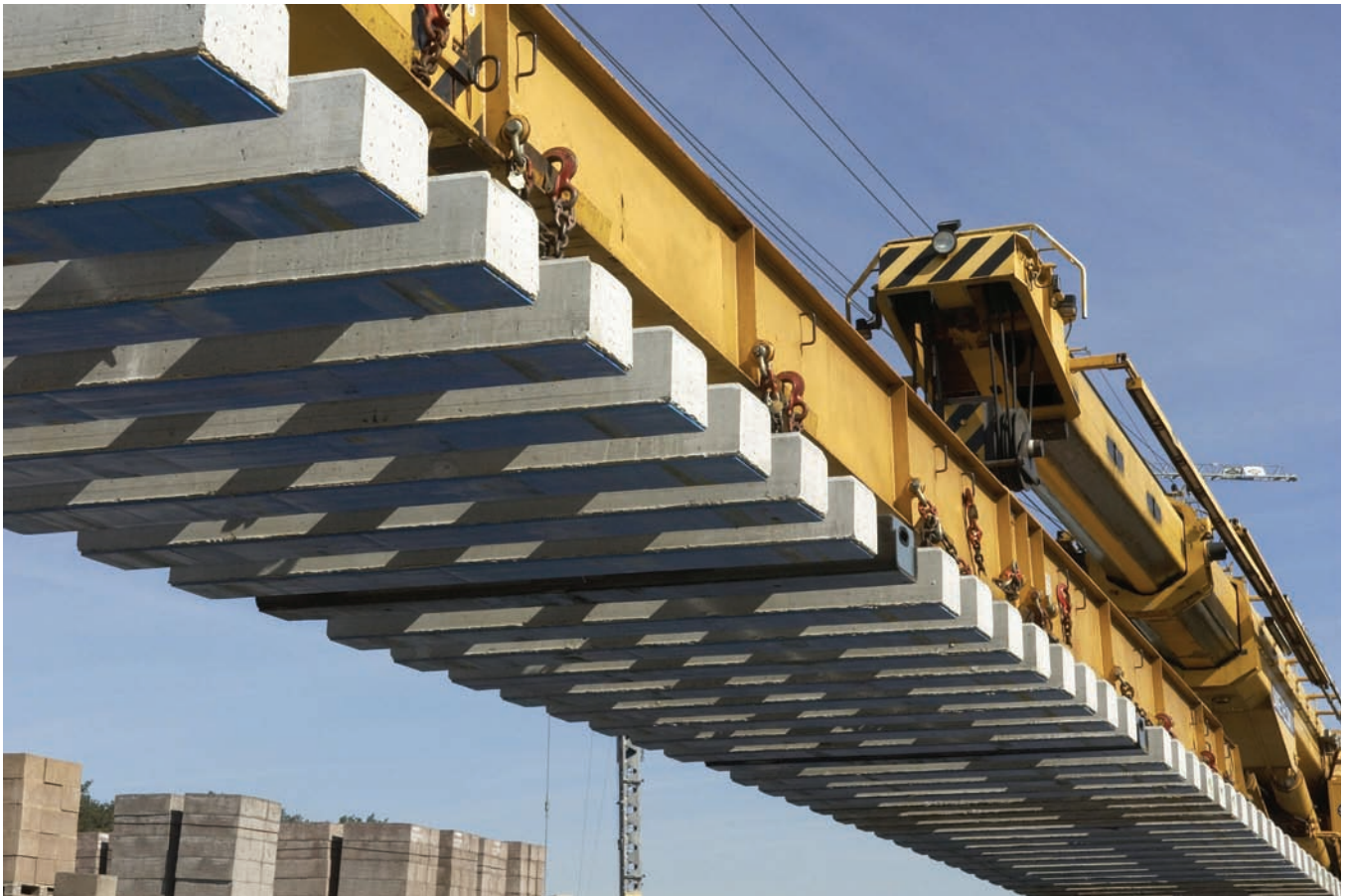
Figure 7: Installation of padded sleepers
