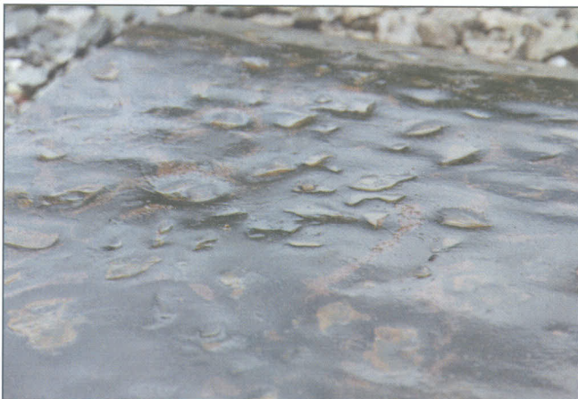
Fig. 3: Ballast grain indentations on the load distribution layer of the ballast mat
