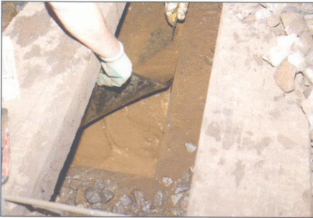
Fig. 2: Presence of water on the tunnel floor
