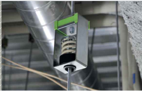
AMC ceiling hangers with Sylomer® bearing
