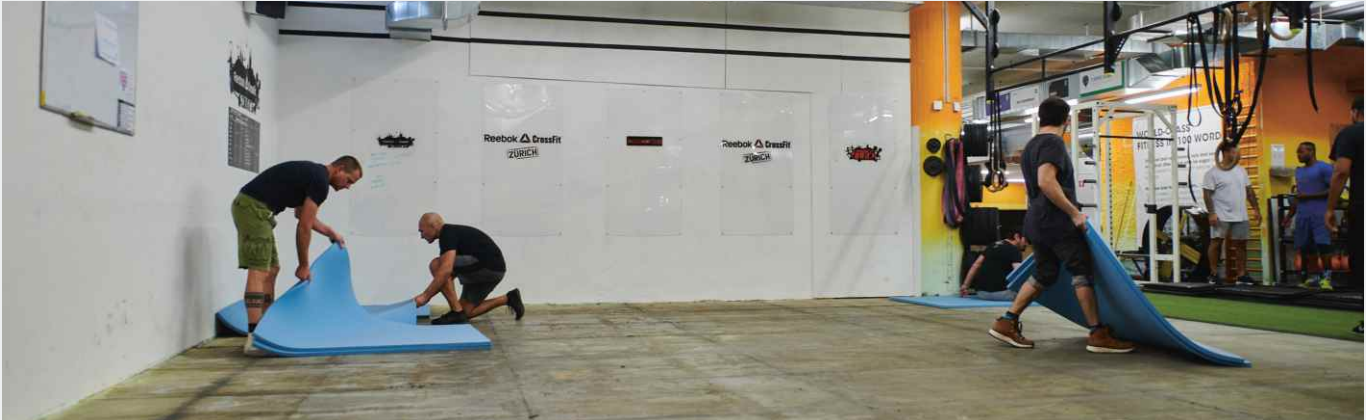
Eric Diaw and team during the installation
